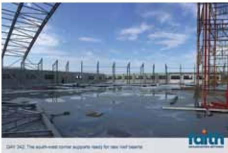
DAY 342: The south-west corner supports ready for new roof beams.
